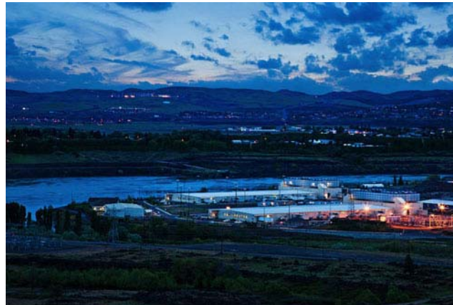
Google data center in Dalles, OR (Columbia river)
